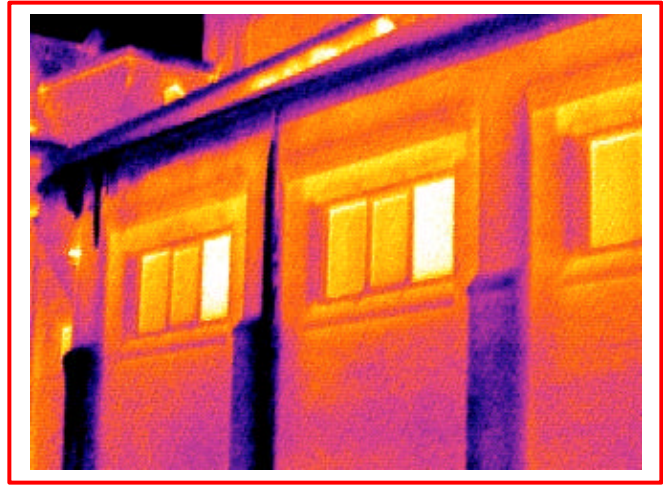
Our Inspection Services Locate the Problem Areas
