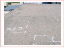
Case Sample: Low-slope roof moisture surveys – IR Inspection by Boldstar moisture infiltration into the roof assembly noted, areas marked & verified
